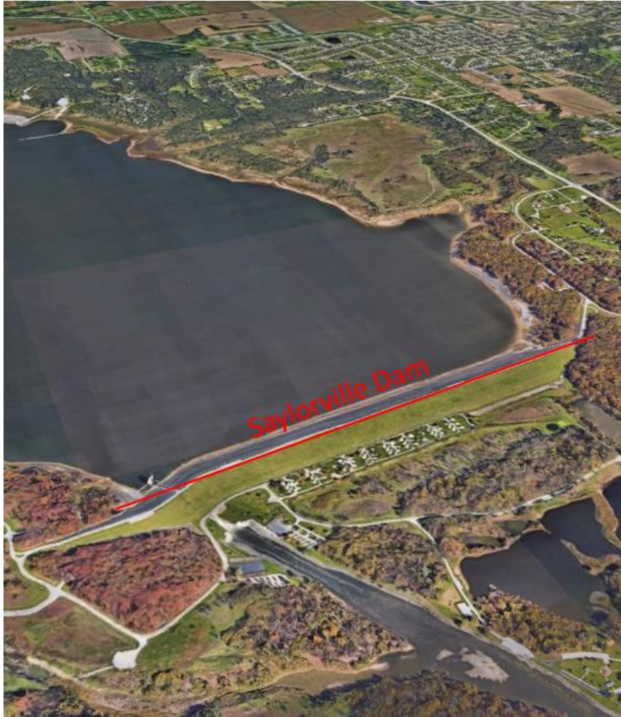
Figure 6.15 Close-up view of the Saylorville Dam.
